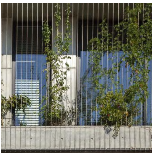
SC-02 - MESH SCREEN (CHARCOAL GREY) TENSILE WIRE BACKING, COLOR TO MATCH MT-04
