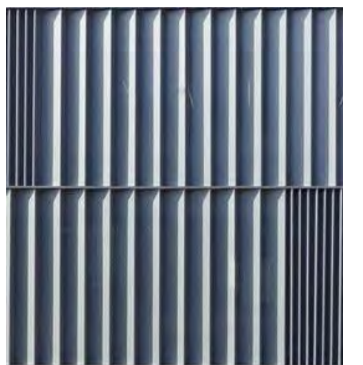
SC-04 - EXTERNAL WEATHER ALUMINIUM LOUVRES (GREY/CHARCOAL GREY) COLOR TO MATCH MT-04
